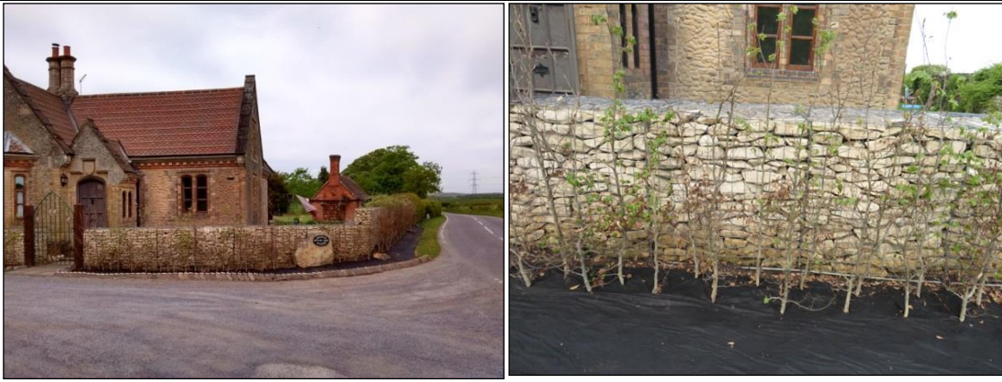
Enclosure including gabion wall with fence panels removed and beech hedge – May 2018
